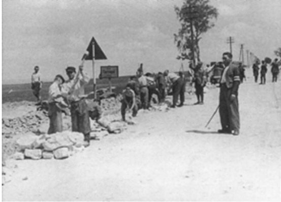
Fig. 13: A Construction Site at the Rollbahn Süd (1942)
